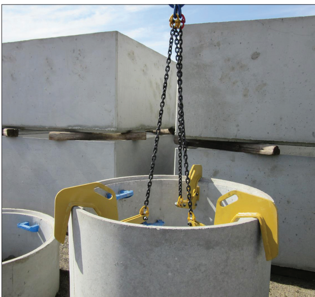
Photo depicting correct lifting gear.
