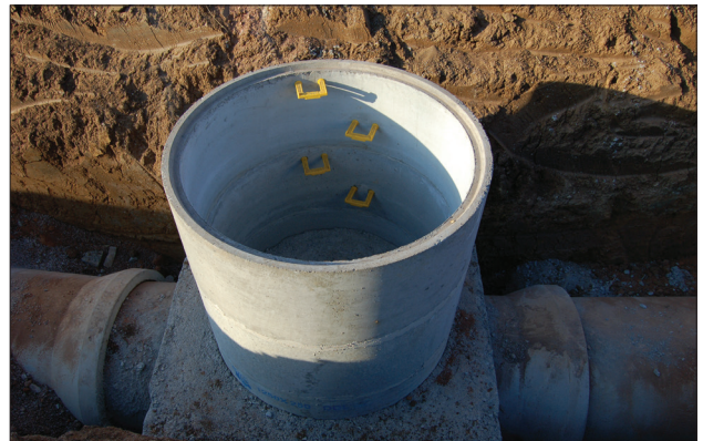
Photo of manhole installed with steps.
