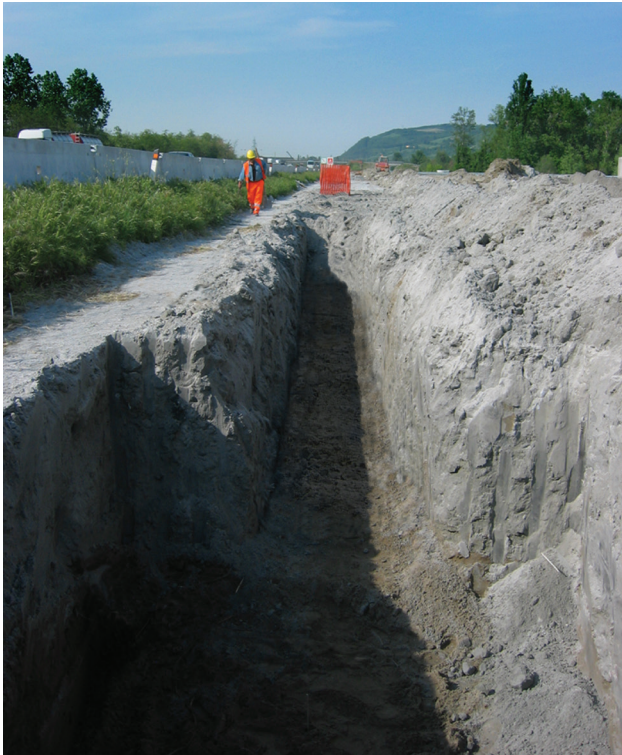
Photo of a well barricaded neat excavation.
