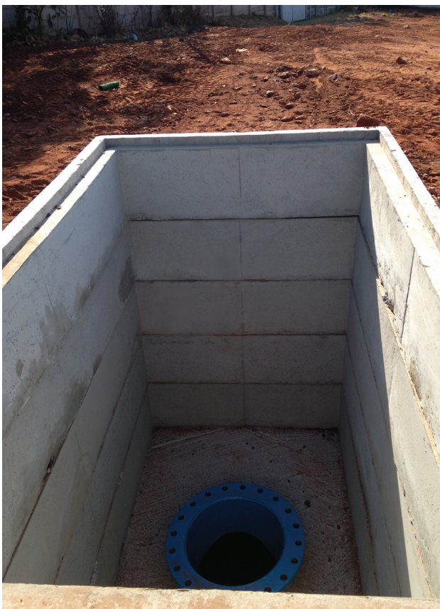
Image of rectangular manhole for valve chambers.
