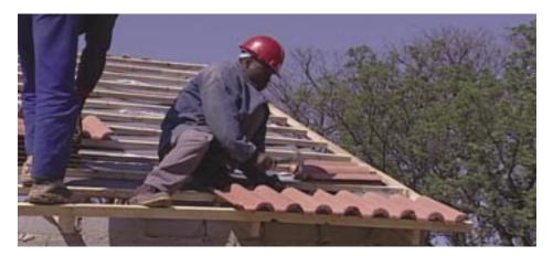
The minimum fixing requirement in unexposed areas is that every tile at the roof overhang and under the ridge must be nailed.
