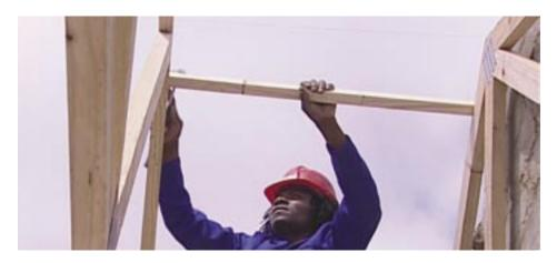
To keep the trusses in a vertical position, 38 x 38 battens are fixed on either side of the ridge.
