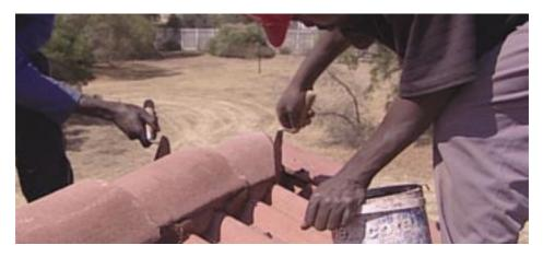
The excess mortar must be cut off and neatly pointed at right angles to the tiling and wet brushed for a neat finish.
