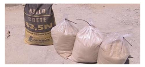
The bedding mortar for bedding of the ridge tiles, consists of 3 parts of clean plaster sand and one part of cement.
