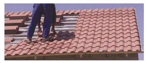
Tiling should always be done from the right to left working from bottom to top in width of three tiles as set out at the eaves and ridges. This is the only way to keep the tiles in a straight line ensuring perfect alignment at the gable ends.
