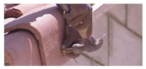
Rake tiles must be fixed with serrated nails.
