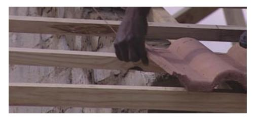
Mark the correct roof overhang with a chalk line from the top batten to the plaster batten.
