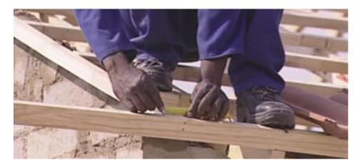
The tilting batten must extend 20 mm past the verge counter batten.
