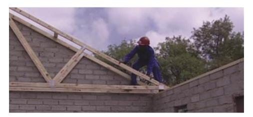
The next two trusses can now be positioned, plumbed and fixed temporarily to the first truss.
