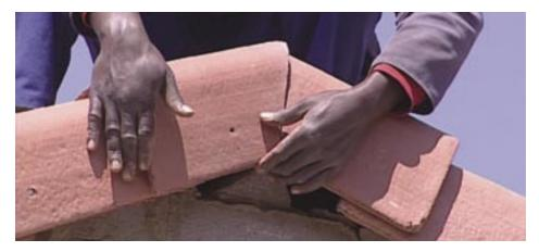
The top rake tiles are mitered on site. Once mitred, top rake tiles form a neat junction on the roof and are bedded with the ridge tiles.
