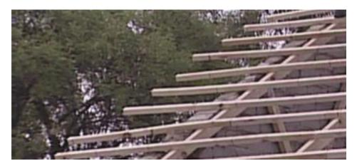
Allow for sufficient overhang at gable ends for trimming.
