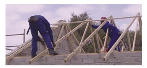
Battens are used as temporary bracing to ensure trusses are installed vertically.
