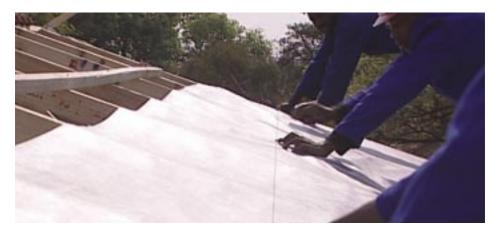
Underlay is secured with clout nails to the centre of the rafters.
