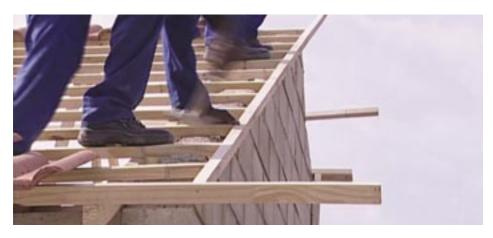
Nail the bottom end to the tilting batten.
