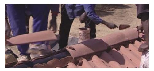
Ridge tiles are edge bedded into a continuous bed of mortar which is placed on top of the top course of tiles.
