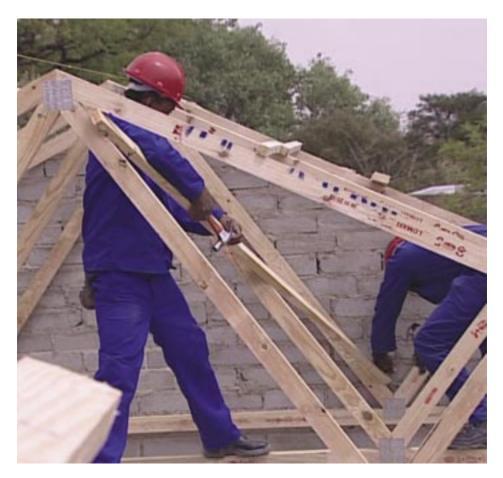
Fix diagonal cross bracing to the long webs of the first three trusses to create a rigid unit to which the other trusses can be attached with temporary battens. These temporary battens and bracing must be removed once all permanent battens are fixed.
