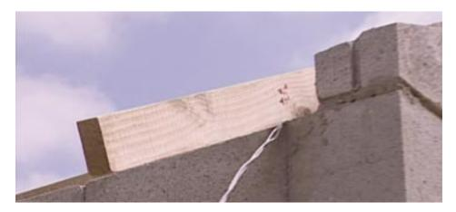
Make sure trusses protrude equally far on both sides over the wall plate.
