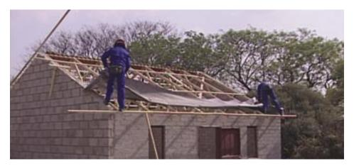
Underlay must be fixed horizontally over the rafters prior to battening.
