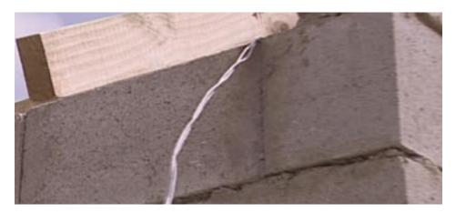
Metal strips or galvanised wires have been built into the wall.
