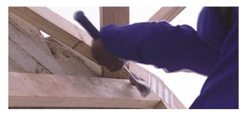
Bracing members must be nailed to the underside of the trusses with 2 nails at approximately a  $45^{\circ}$  angle from the apex of the truss to the heel of the truss.
