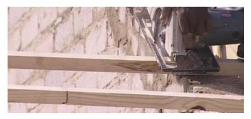
Cut off the end of the tiling battens, but do not cut the bottom tilting batten.
