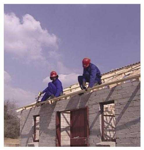
Fix a 38 x 50 mm tilting batten placed on edge flush with the ends of the rafter.
