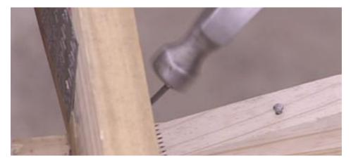
Bracing members must be connected to the wall plate with 3 nails.
