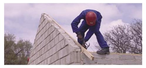
Nail trusses to wall plate.
