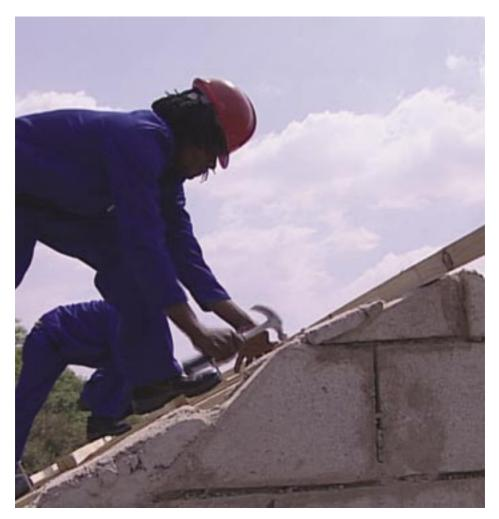
Place the top tiling batten maximum 25 mm away from the apex (top end) of the trusses and nail into position.
