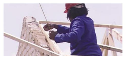
Mark the batten centres at each end of the first and last truss.
