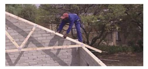
Adjust position of first and last truss at gable ends to ensure equal spacing at gable walls.
