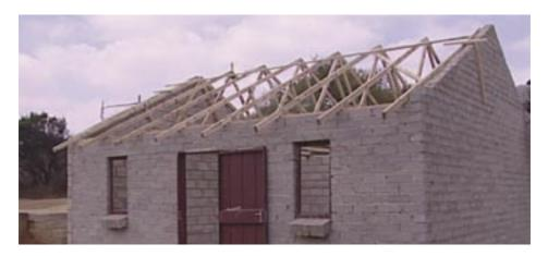
The remainder of the trusses can now be erected and attached to the three braced trusses.
