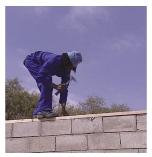
Align wall plate minimum 76 x 38 mm with inside wall and nail into position using 75 mm wire nails every 400 mm along wall plate.
