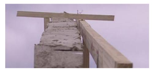
Position first and last truss using temporary support bracing.
