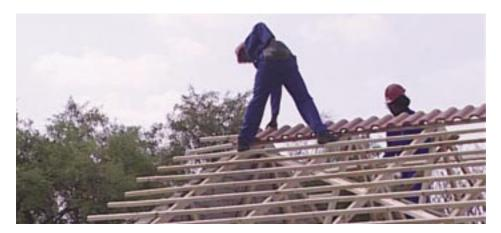
Adjust tiles to ensure that an equal roof overhang is achieved at both gable ends with full tiles.
