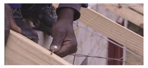
Span a fish line above the wall plate from the first to the last truss to check alignment.
