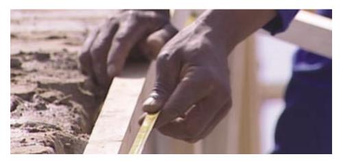
Measure 335 mm from the top of the first tiling (plaster) batten down the slope of the rafter and make a mark on the first and the last rafter.
