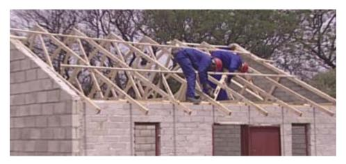
Permanent diagonal bracing must now be installed at one gable end of the roof. Bracing members must be a minimum of 38 x 76 mm.
