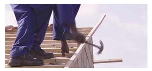
Nail the verge counter batten to the ends of the tiling battens at both gable ends.
