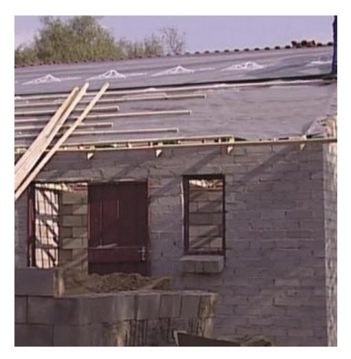
At open eaves, the underlay can be stopped for aesthetic reasons at the external wall protruding the outside wall face, by 20 mm.
