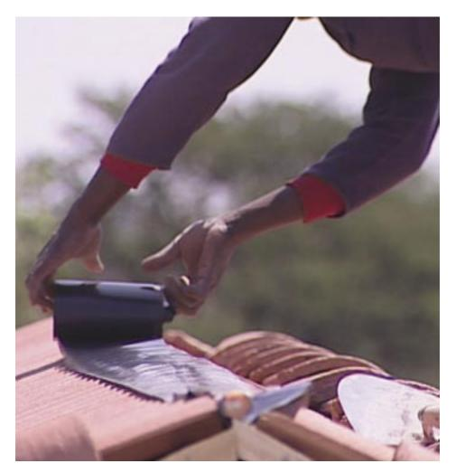
Before bedding, a 150 mm wide DPC must be installed under the ridge tiles.
