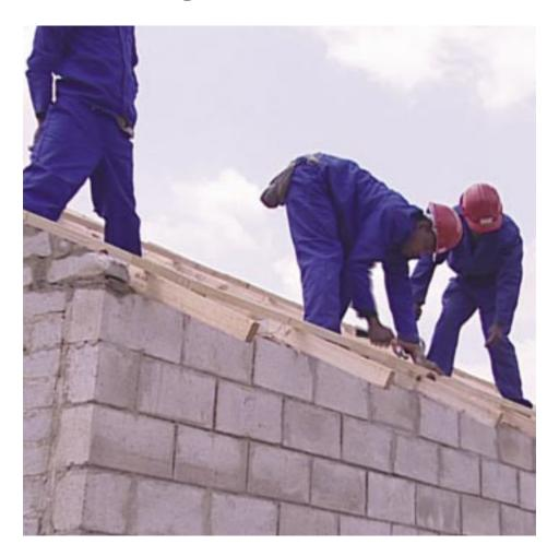
At a one tile roof overhang at eaves, place the first tiling batten (plaster batten) in line with the outside wall so that it acts as a finishing batten for plastering the outside wall.
