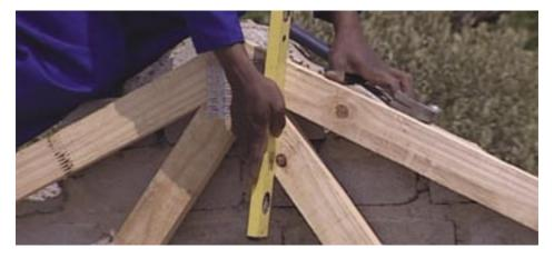
Make sure trusses are plumb (vertical).
