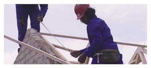
Measure the distance from the top tiling batten to the top of the plaster batten. Divide equally by the number of courses required to establish the correct batten centres which should be between 320 and 345 mm.
