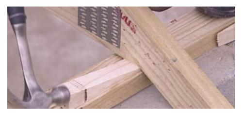
Adjust if necessary with wooden wedges under the tie beams of the trusses.
