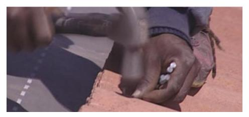
Clout nails must penetrate the batten by at least 25mm (75mm long nails for Double Roman tiles).
