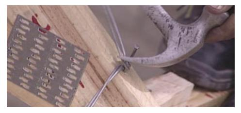
To resist uplift forces, each truss must now be permanently anchored to the wall and wall plate with these metal straps or galvanised wires.
