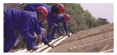
Fix battens with 75mm long nails according to chalk lines. Battens must span over at least 3 trusses and the joints must be staggered.
