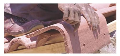
Mark the front of the first rake tile and cut to line up with the eaves course of tiling. The first rake tile must butt up against the second course of tiles.
