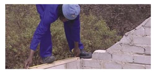
Mark position of all trusses at max centres of 900mm on both timber wall plates.
