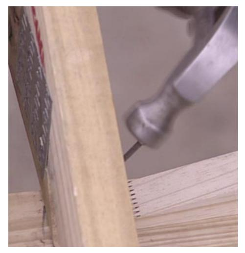
Scew nail all trusses with 100 mm nails to the wall plate.
