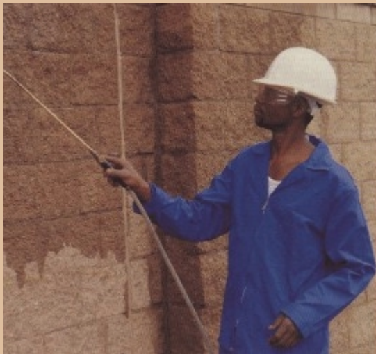
Applying sealers to masonry wall
