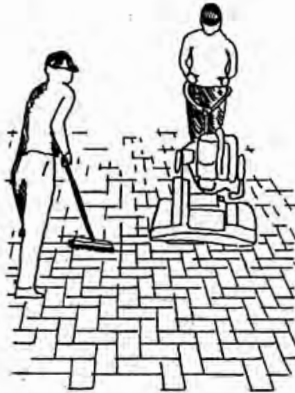
Joint filling and final vibration
